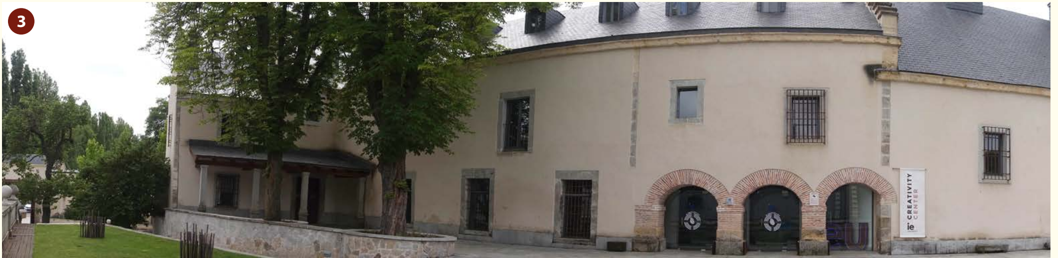
The large L-shaped building complex where the delivered metal was processed. Photo: UK.
